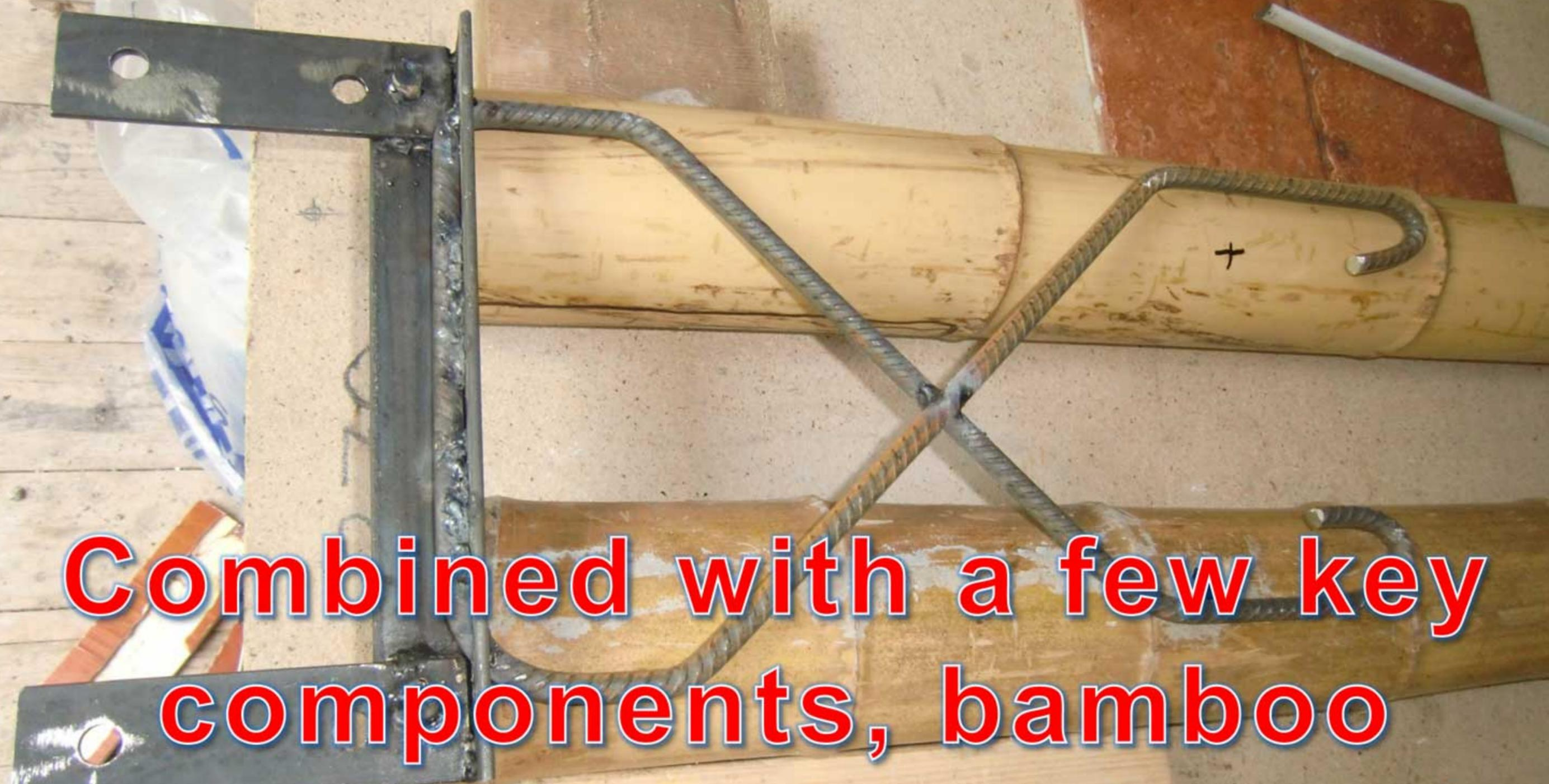
**Combined with a few key components, bamboo provides earth quake safe connections**
